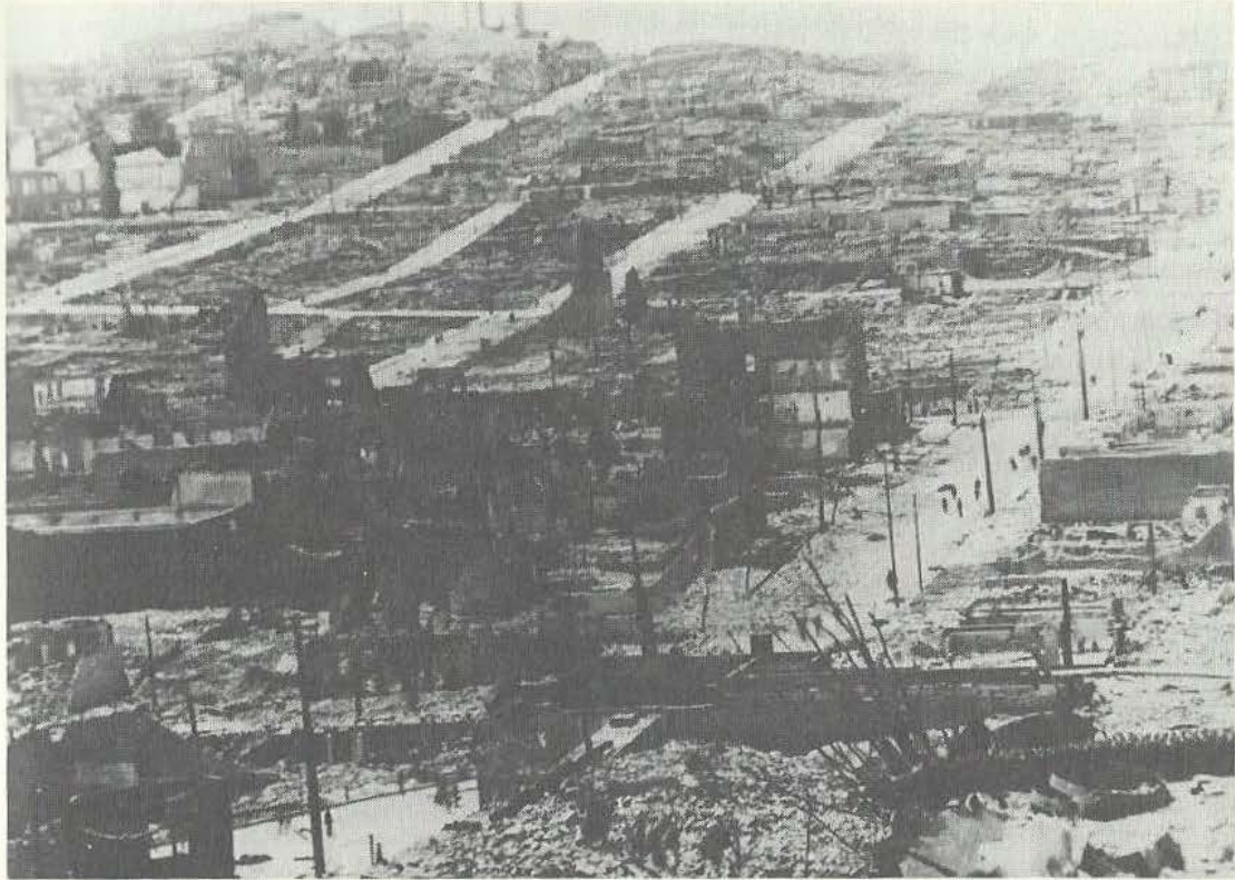
Only a fifth of the total destruction was caused directly by the earthquake; the rest came from the ensuing fire.
