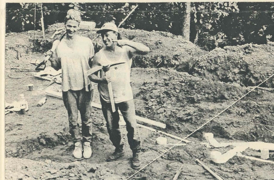
Jessy Lynn Smith & Angela Brightfeather laying pipe
